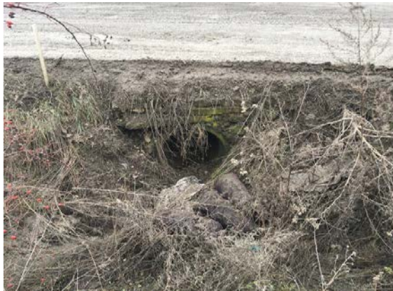
View of inlet
