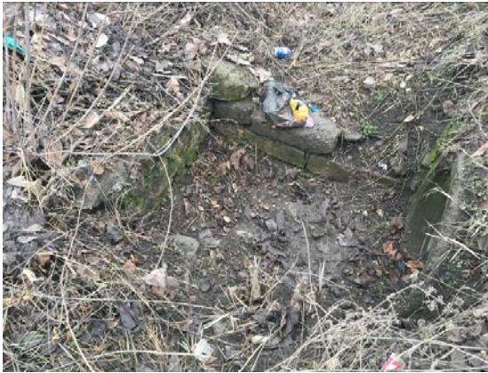
View of inlet
