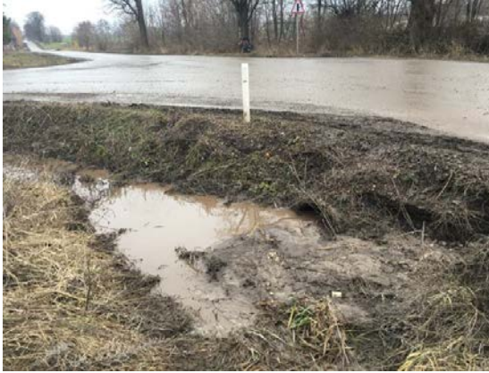
View of inlet
