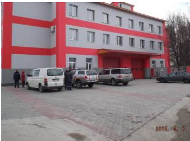
Typical required pavement with interlock bricks in combination of 2 colors. Picture from NAVFAC project completed in Balti (Moldova).
