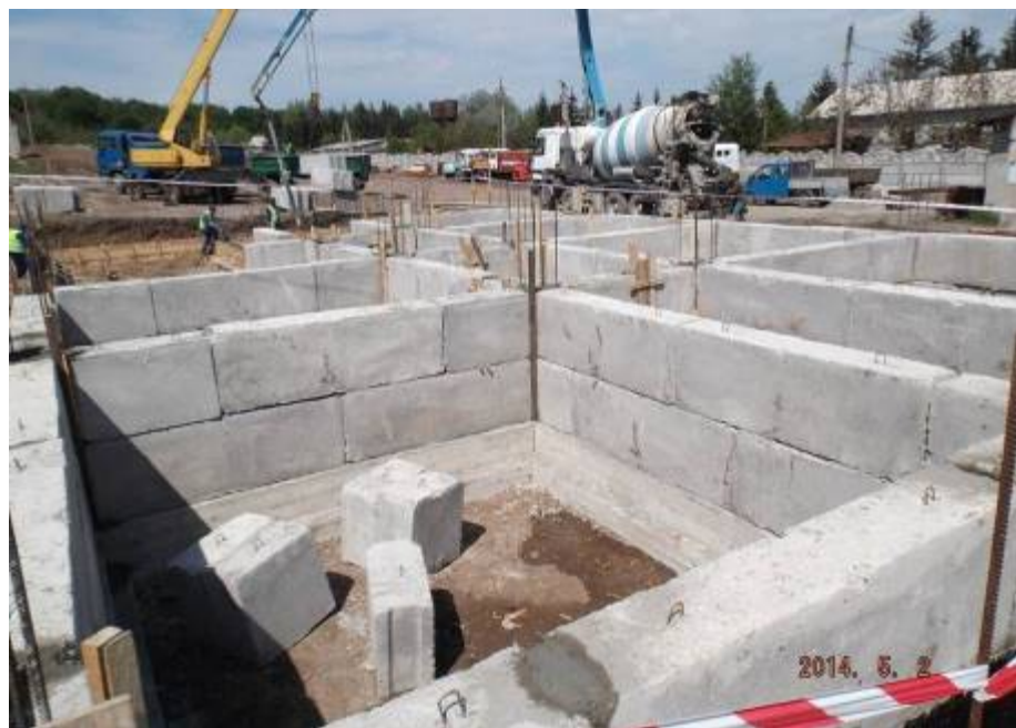
Typical concrete block foundations required due to high seismic requirements for a similar new Fire and Rescue Station built in Moldova.
