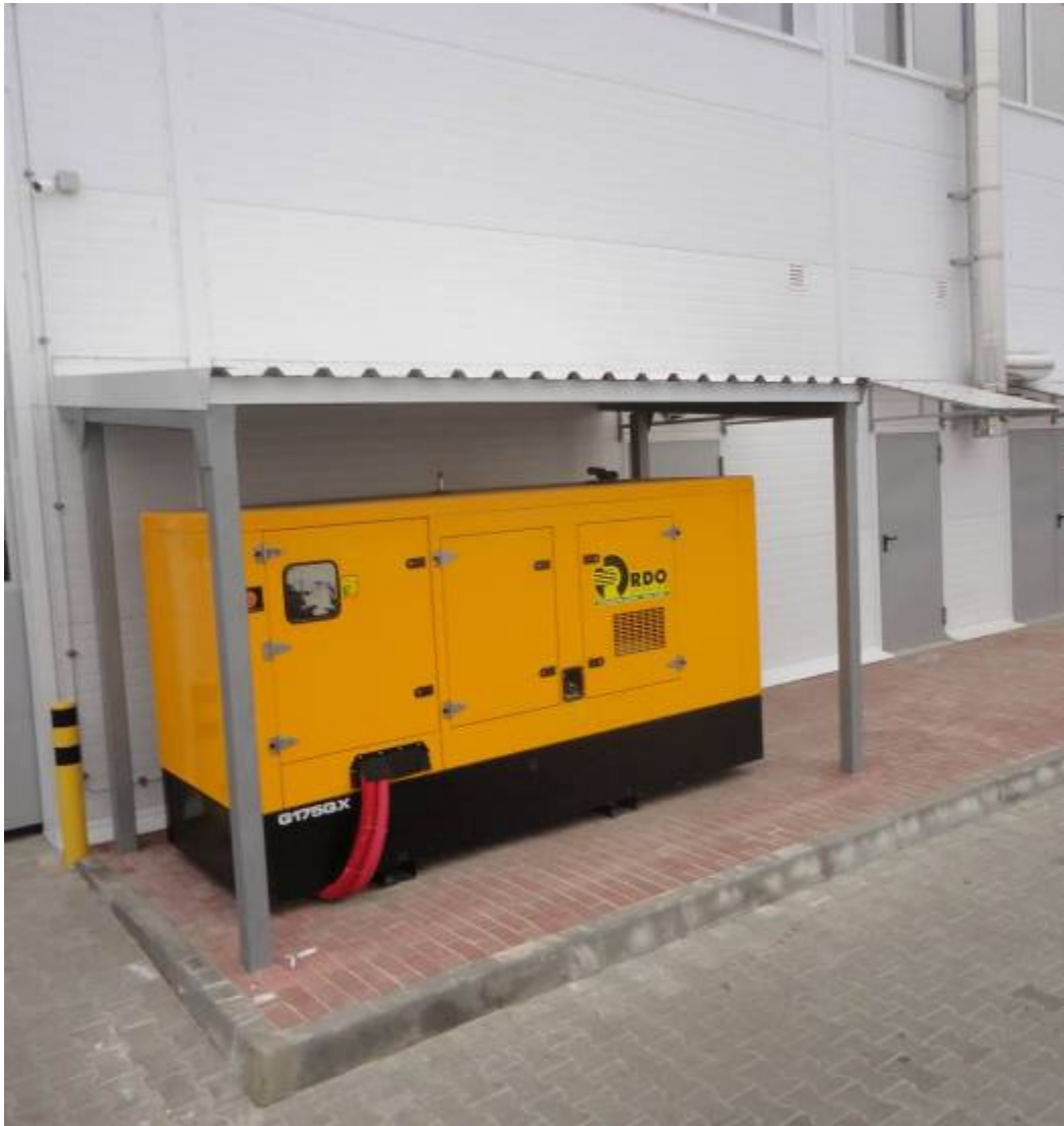
Typical acceptable type of exterior generator, under a light metal canopy. The one required in our project shall be relatively larger than the one shown in the picture, from a recently completed project in Ukraine
