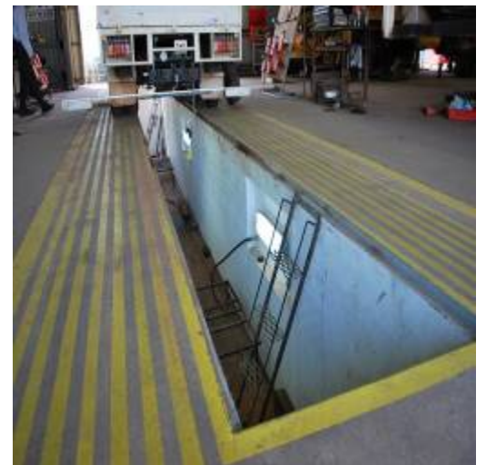
Typical maintenance pit. Provide with very high illumination level (explosion proof equipment)
