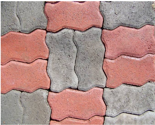
Typical installation of interlock bricks
