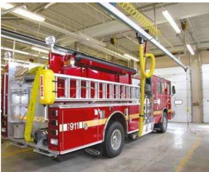
Typical hose exhaust extraction system
