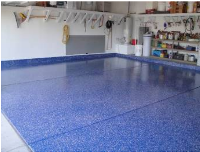
Typical epoxy cover for concrete
