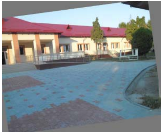
Typical required pavement with interlock bricks in combination of 2 colors. Picture from NAVFAC project completed in Romania.
