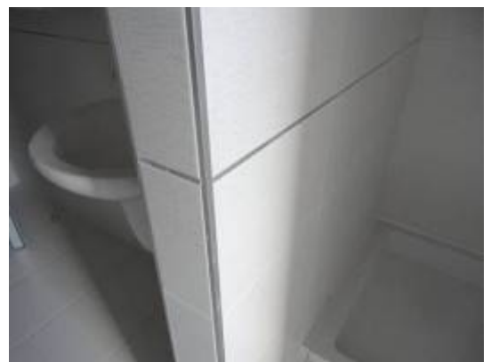
Typical required level of quality for the toilet ceramic tiles on the wall. Provide stainless steel or aluminum corner protection. The use of plastic corner guards is not authorized.
