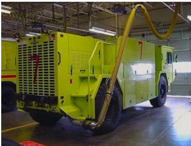
Typical hose exhaust extraction system
