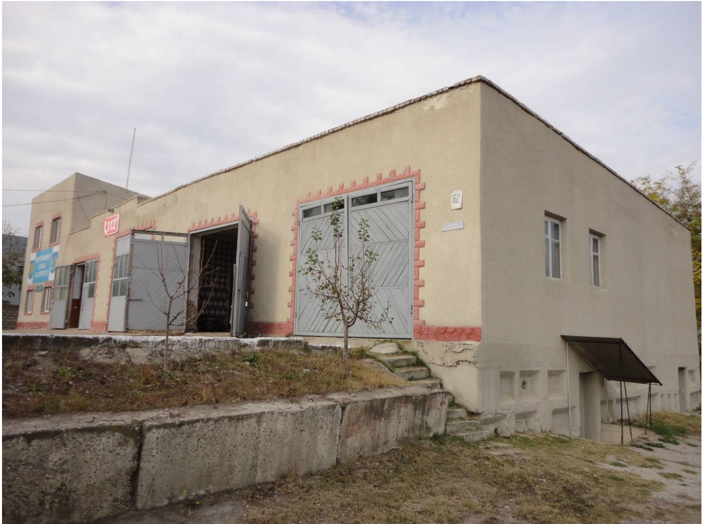
Building to be completely demolished. Note the existing retaining walls to allow for leveled area in front of the truck bays and sloped road towards the back of the building. The draft conceptual designs included in this document follow the same concept, to provide retaining walls around the plot of land
