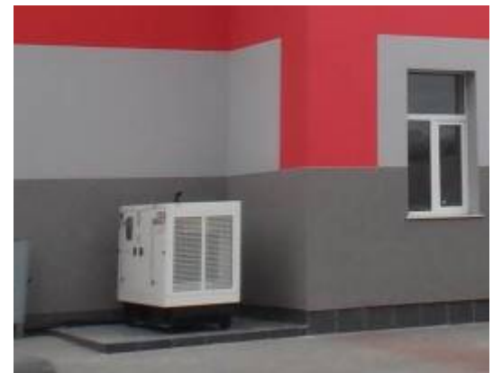
Typical pad mounted generator installed in Balti FRS by NAVFAC. In Anenii Noi it shall be provided with an additional weather protection.
