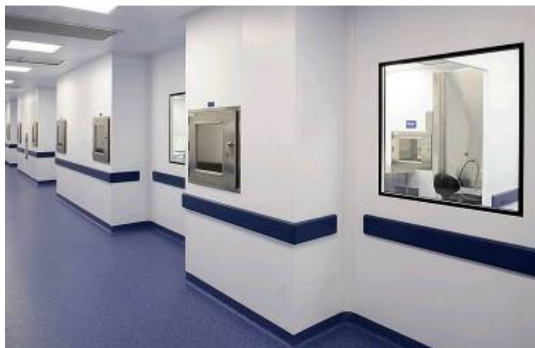
Typical required PVC wall protection
