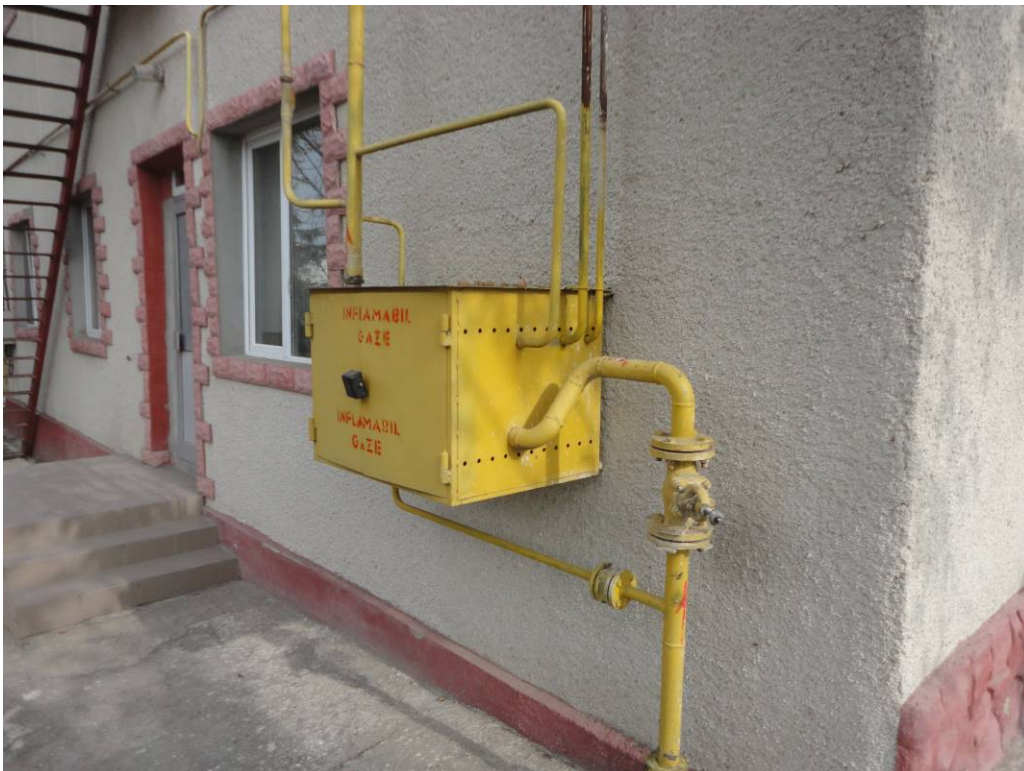
Gas installation to be removed in coordination with the gas supply company. All equipment to be reused if allowed and approved in writing by the gas supply company.
