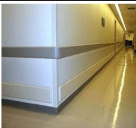
Typical required PVC wall protection
