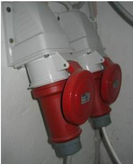
Typical required IEC-60309-style plugs inserted into wall-mounted sockets
