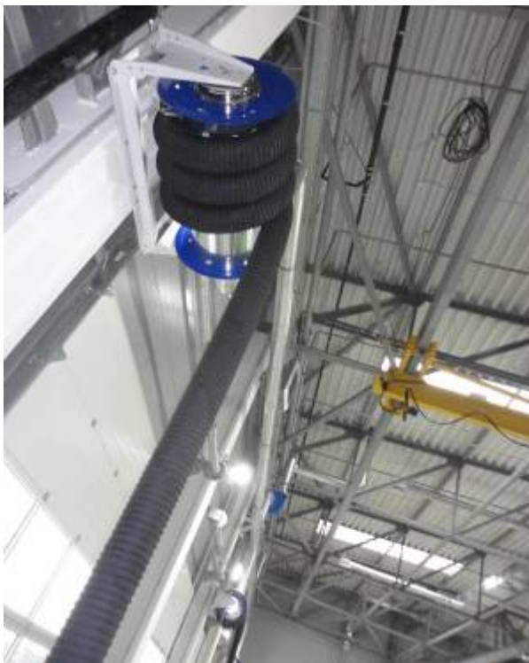
Hose extraction system for fumes in recently completed project in Ukraine
