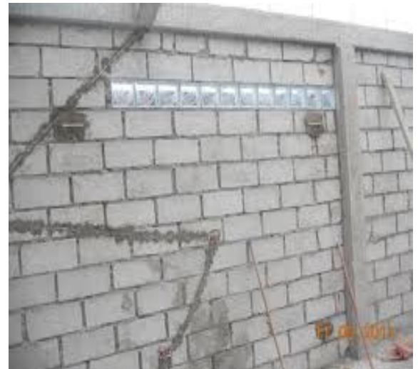
Typical electrical conduits within walls
