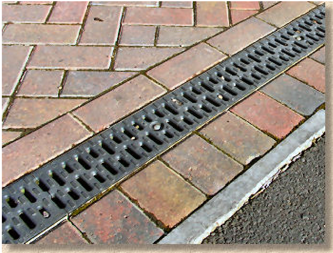
Typical drainage channel required at the pavement outside the truck bays
