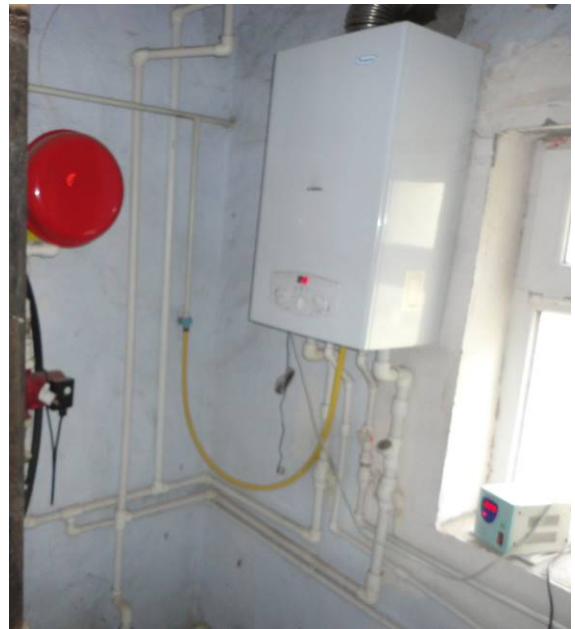
For estimating purposes: The Contractor can estimate that they can use the existing boiler and some piping, but supplemented by another one to be installed in parallel. The Contractor shall reutilize anything that can be reutilized in compliance with Moldovan regulations.
