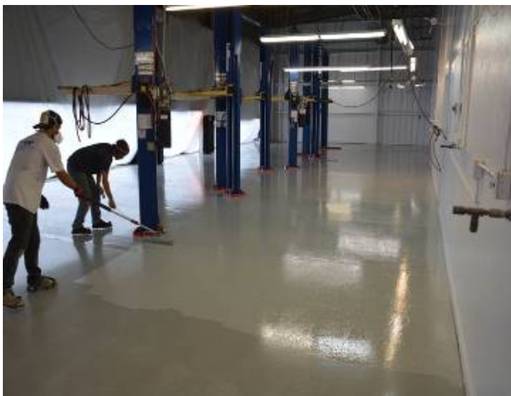
Applying epoxy treatment to concrete flooring. Flooring shall be perfectly leveled prior to the installation of any final layer.
