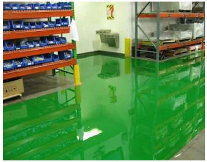
Typical epoxy cover for concrete in green color, as required by our contract.
