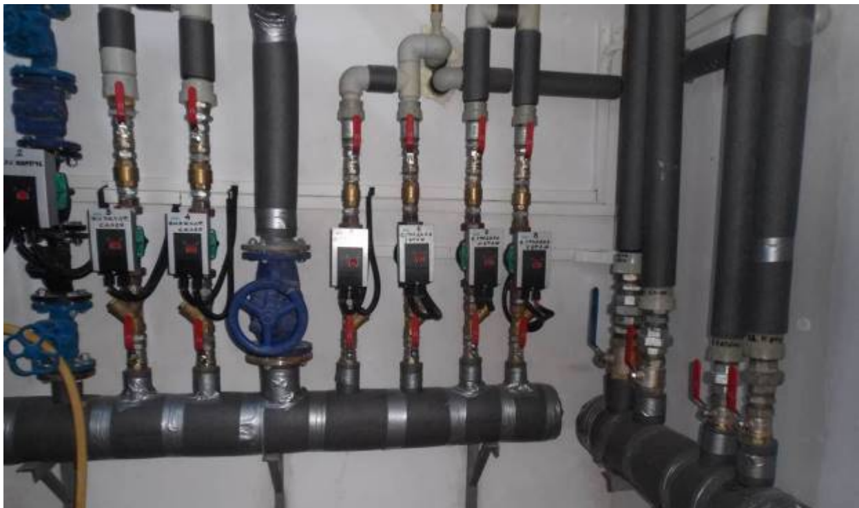
Manifold and dual pumping system from NAVFAC contract in Bulgaria (different loops as required in Anenii Noi)
