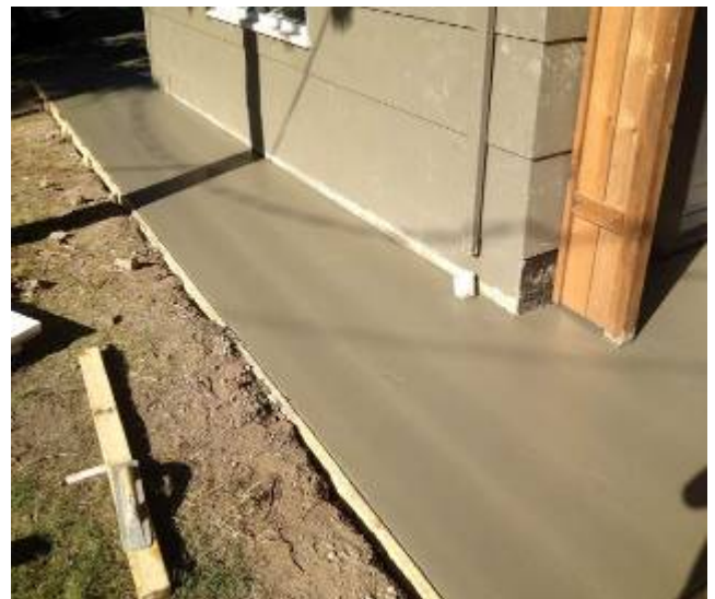
Concrete sidewalk after pouring concrete.
