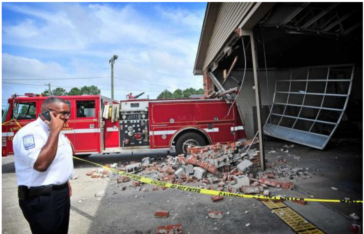
Example of accident for not having bollards at the entrance of the truck bays
