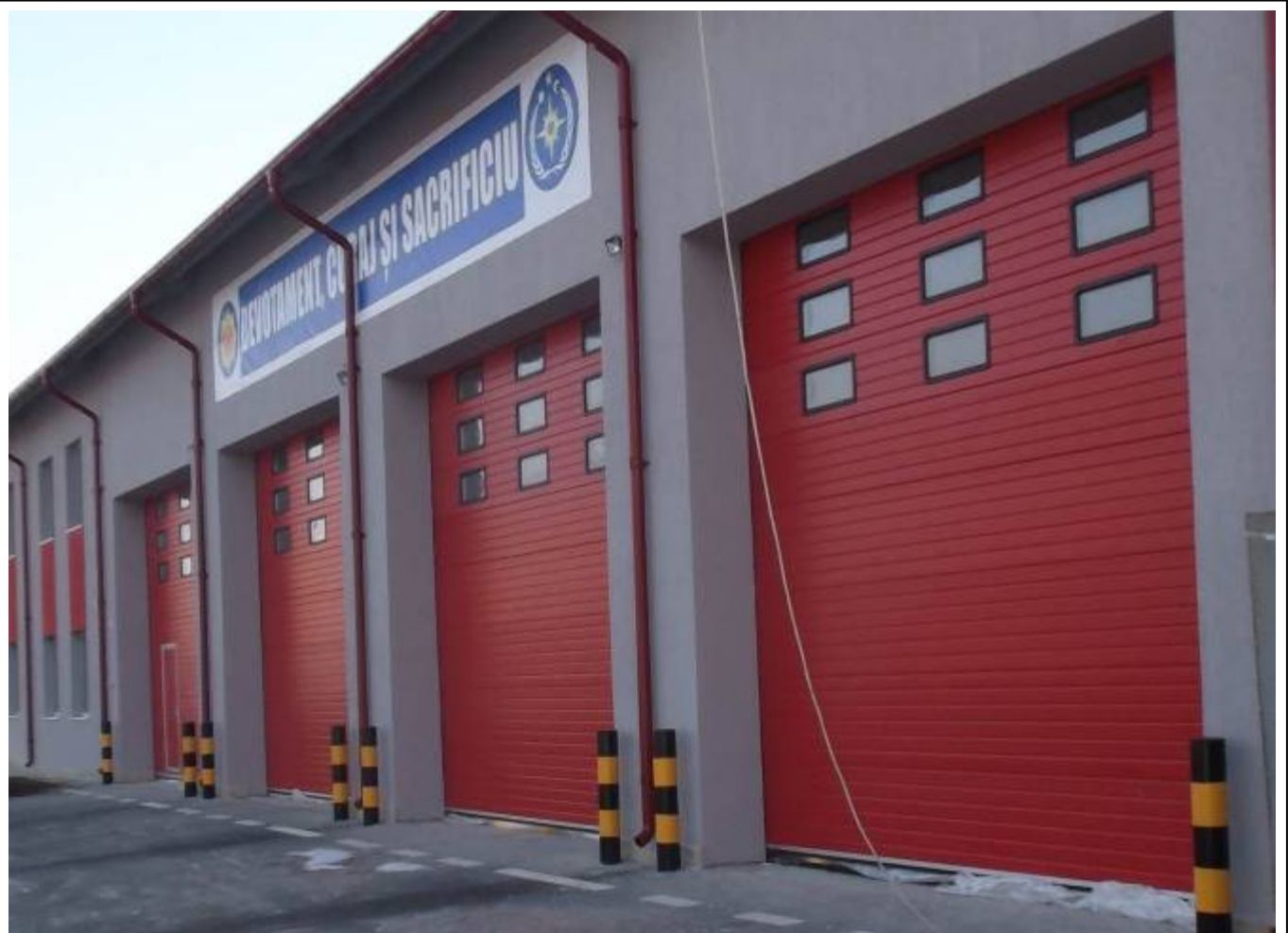
Typical required roll up doors from new FRS built by NAVFAC in Moldova. Notice pedestrian door in the roll up door to the left
