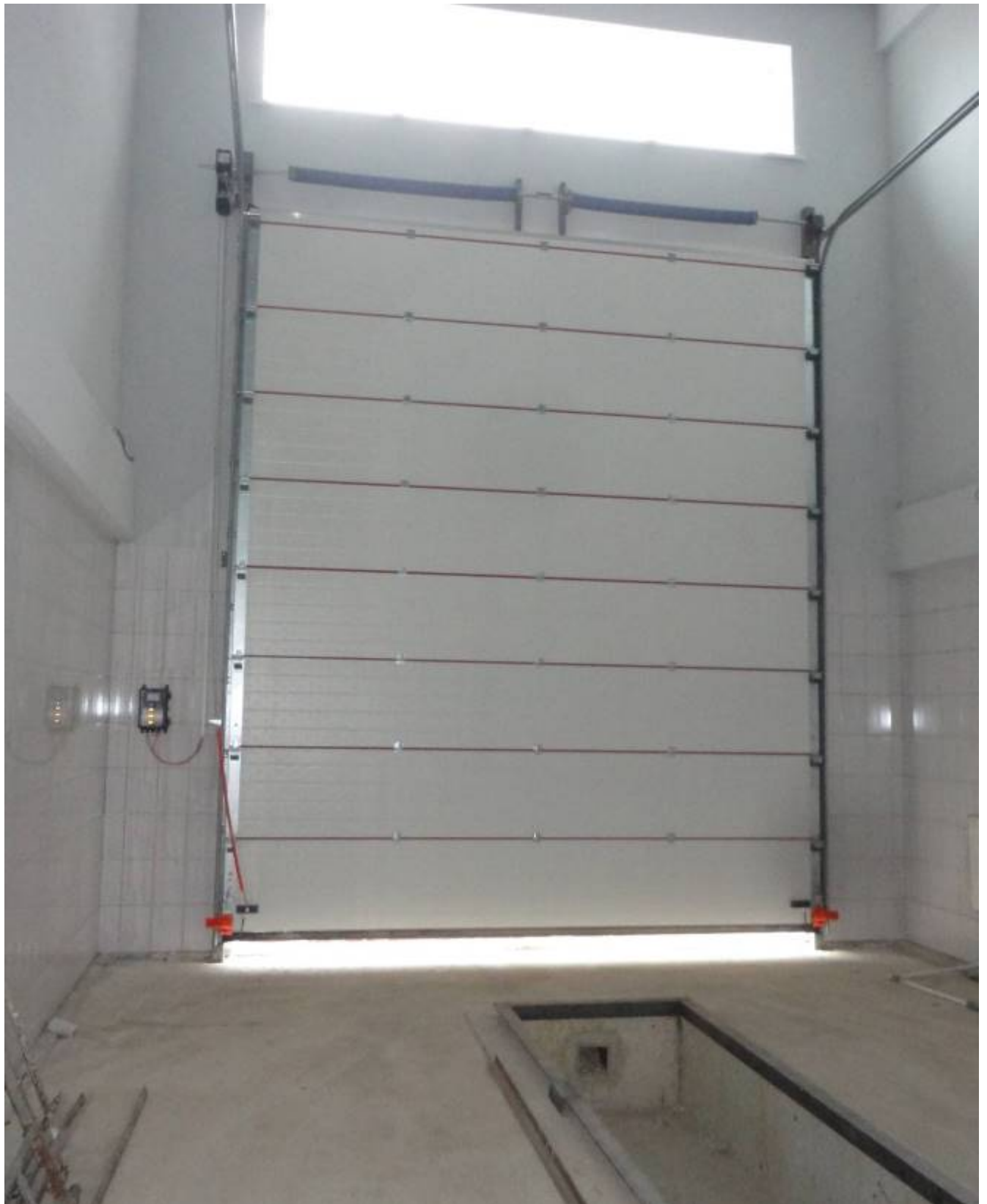
Typical required roll up doors from new FRS built by NAVFAC in Moldova. Notice windows above the door, which is also acceptable. See the drainage sump pit (under construction) to capture the water from washing the fire trucks
