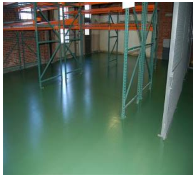
Typical epoxy cover for concrete in green color, as required by our contract.
