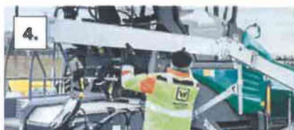
Suspend the extension beam.
