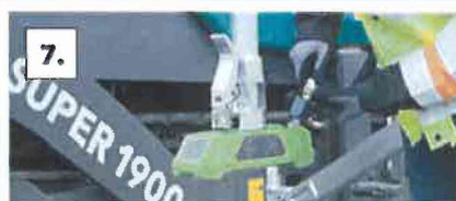
Route cables and connect sensors.
