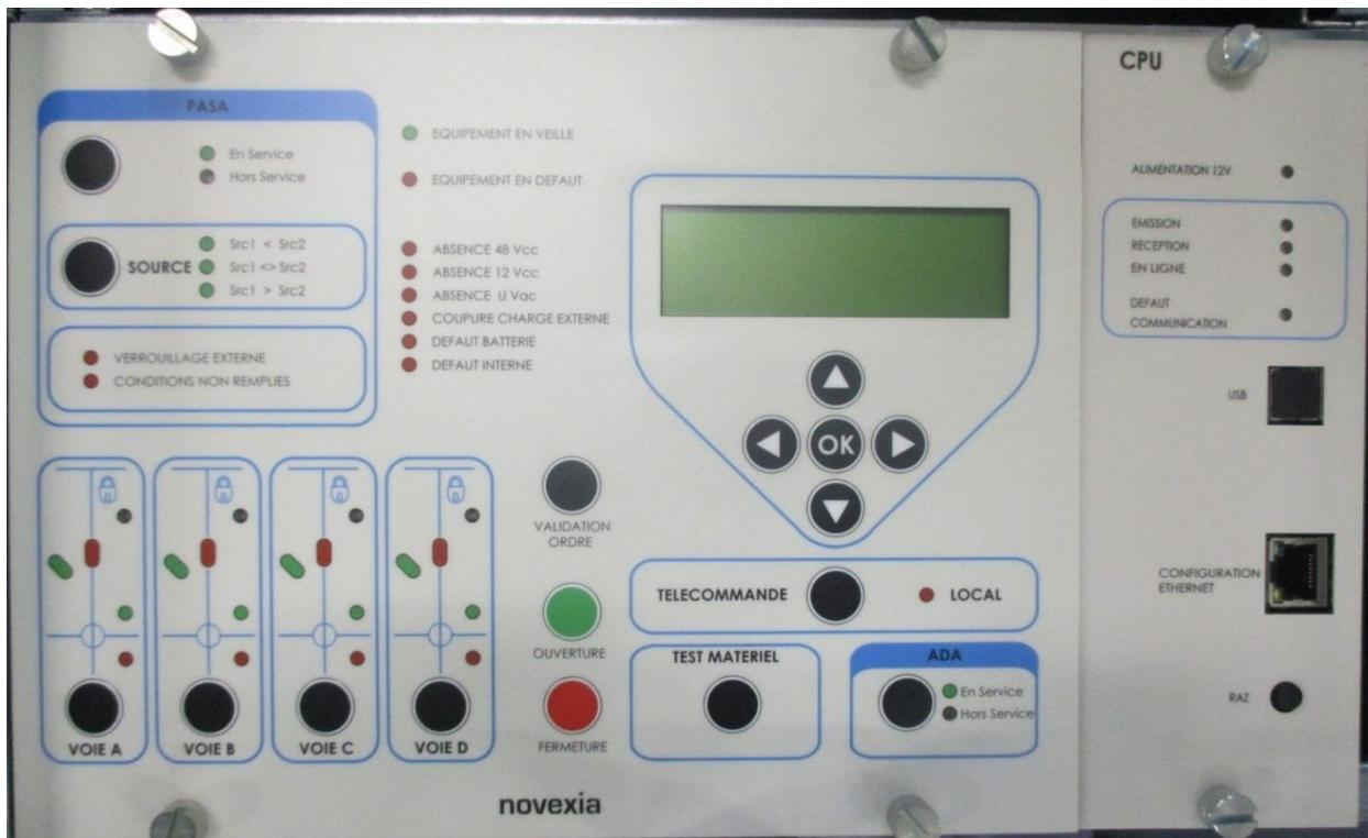
Press the **EQUIPMENT TEST** button and check that all the indicator lights come on and that the display is off.
