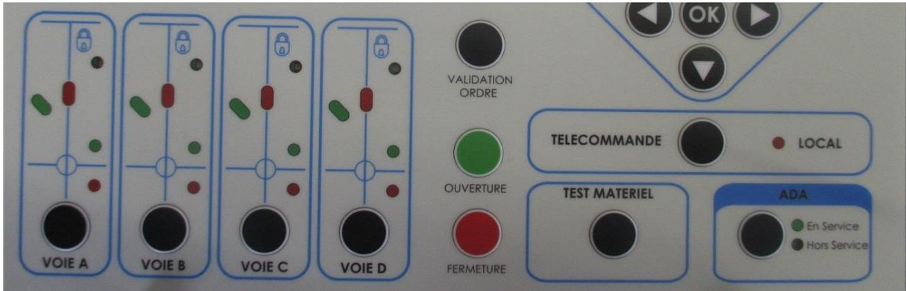
To close a channel, first select the channel to close, then press the "CLOSE" and "COMMAND VALIDATION" buttons at the same time. After closure, the red position indicator lights up
