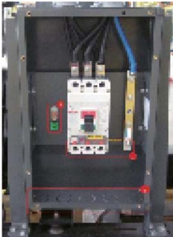
Figure 3.2 Gen-set field wiring of load cables
