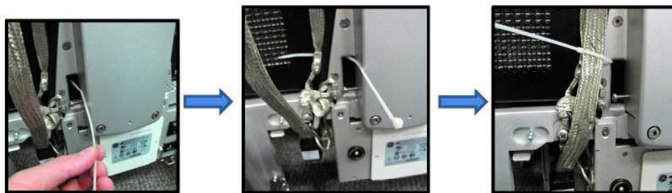
Figure 8-8. Add lower cable tie
