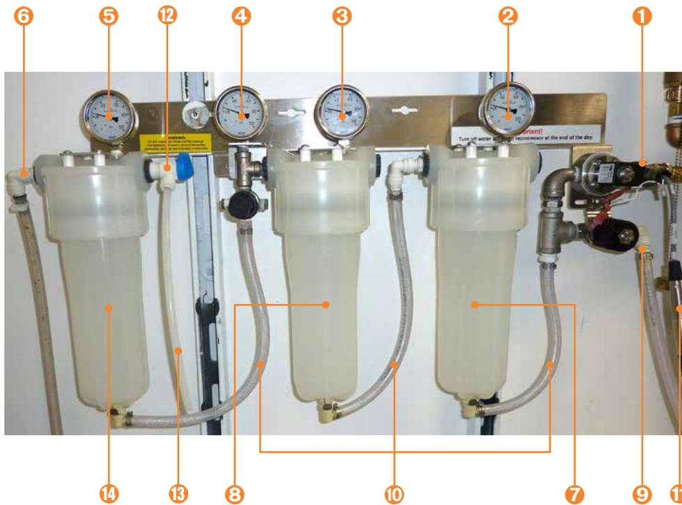
**Figure 4 Water Filtration System**
