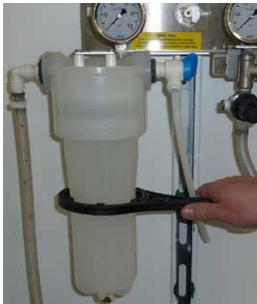
**Figure 7 Loosen Filter Housing**
