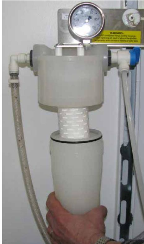
**Figure 8 Remove Housing and Filter**
