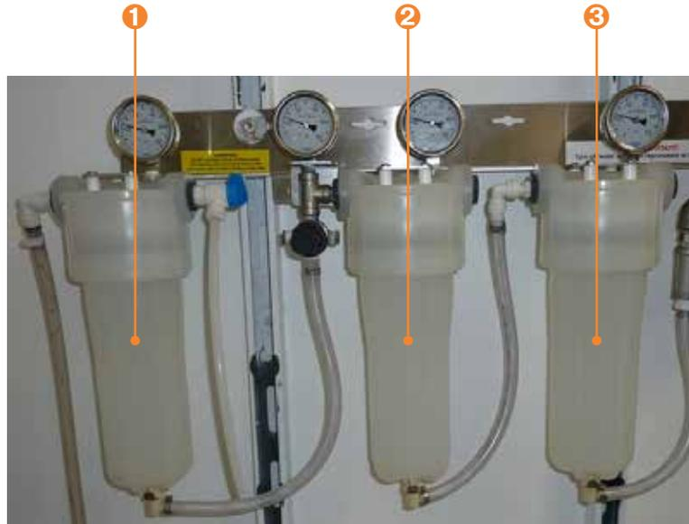
**Figure 6 Filter Cartridges in Place**
