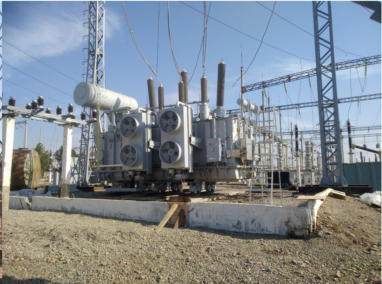
Uzbekistan HV Dual Voltage Transformer 220-110/35kV 63MVA
