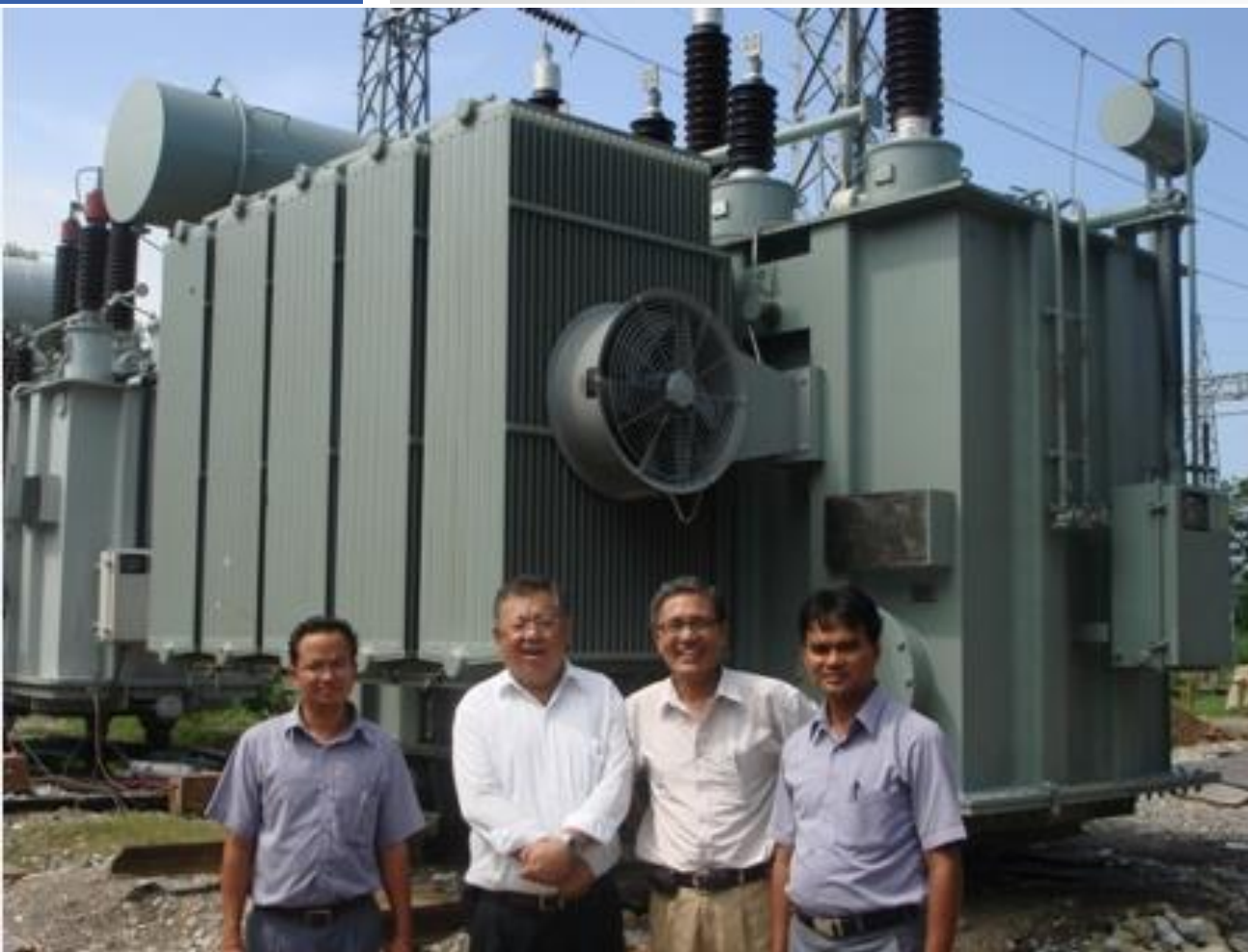
Nepal Electricity Authority 132kV 63MVA power transformer
