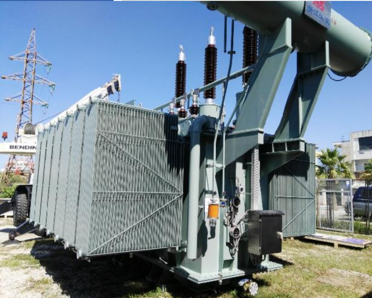
Albania 115kV 31.5MVA power transformer
