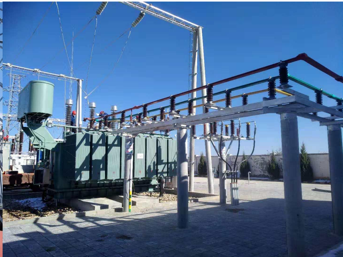
Shaanxi Geopower 110kV 31.5MVA power transformer
