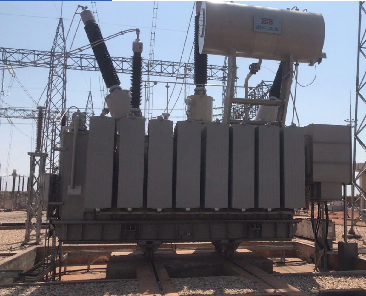
Rwanda HV Dual Voltage Transformer 220-110/33kV 20MVA
