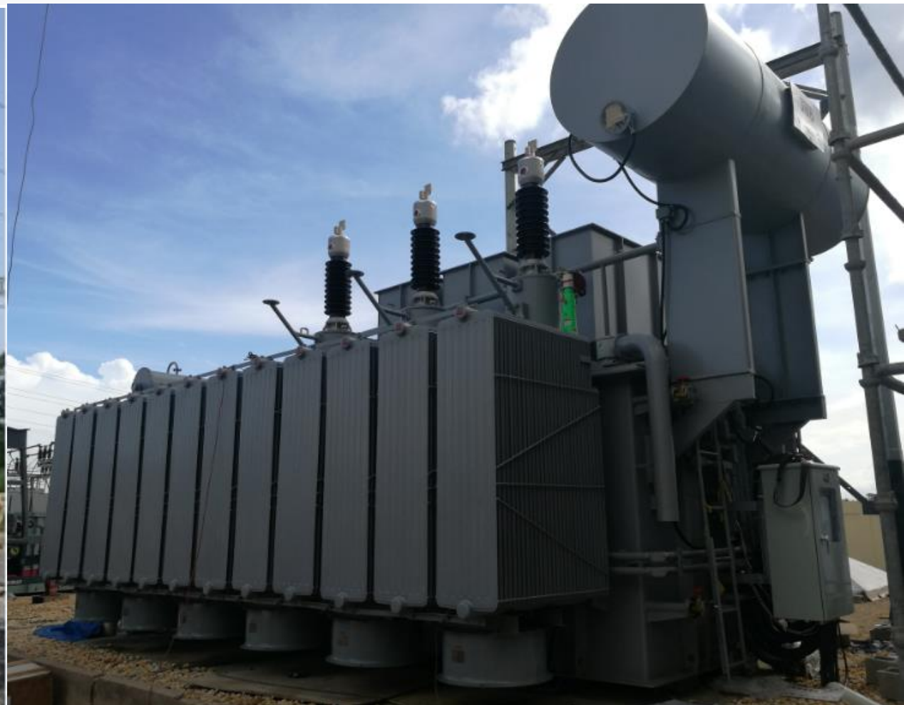
Trinidad & Tobago Electricity Commission 66kV 130MVA power transformer
