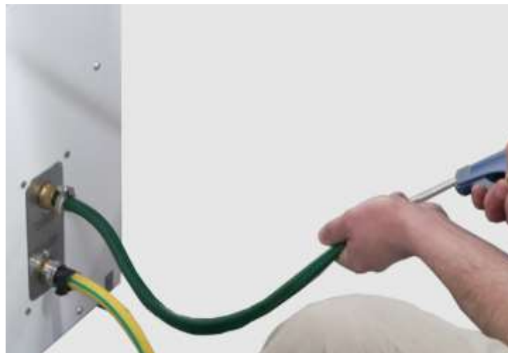
Fig. 32: Purging the cooling water from the system with compressed air
