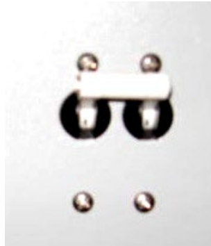
Figure 6: Circuit Breaker Up
