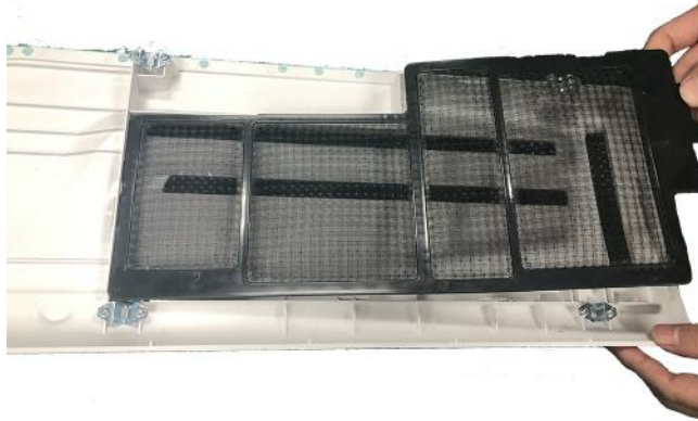
Figure 4-27. Remove the Filters
