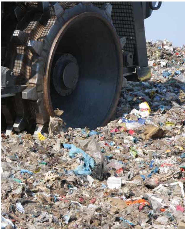
Scrapers ensure clean wheels and high compaction.
