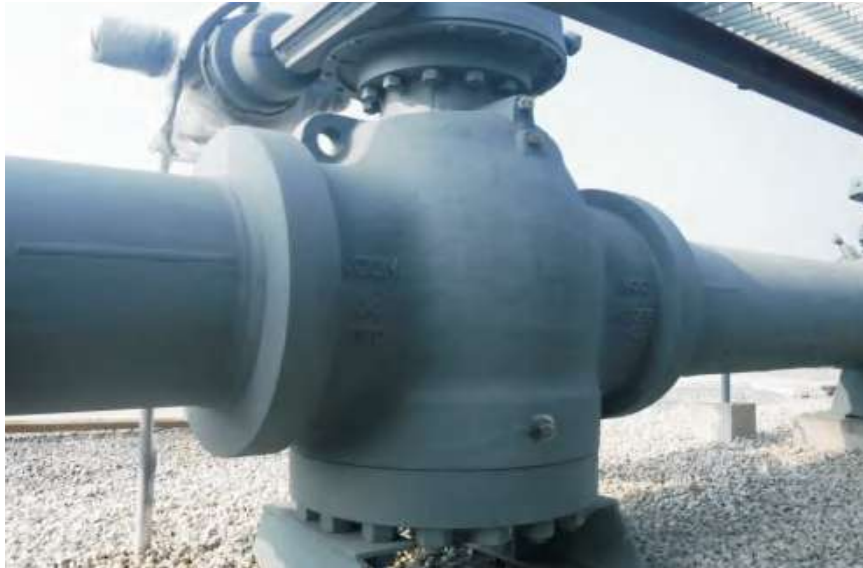
24"-Class900压力平衡式油密封旋塞阀2018年应用在中国石化鄂安沧天然气管道项目 24"-Class900 Lubricated Pressure Balance Type Plug Valve for Sinopec Erdos-AnPing-CangZhou Natural Gas Pipeline Project in 2018.
