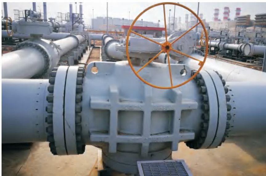
36"-Class600压力平衡式油密封旋塞阀2017年应用在埃及天然气发电厂 36"-Class600 Lubricated Pressure Balance Type Plug Valve for Egyptian Natural Gas Power Plant in 2017
