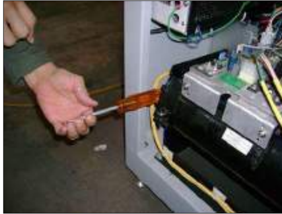
Figure 194: Using Screwdriver to Move Generator
