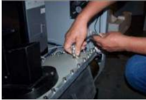
Figure 205: Removing Generator Mounting Bolts
