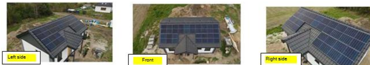
fig.5 Example of photovoltaic installation photo documentation - REQUIRED BY THE MANUFACTURER
