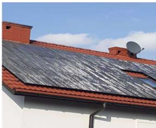
fig.1 LRF effect on a sunny day
