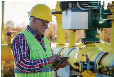
▲ Fuel supply inspection
