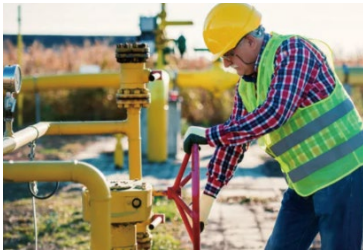
▲ Gas pipeline inspection
