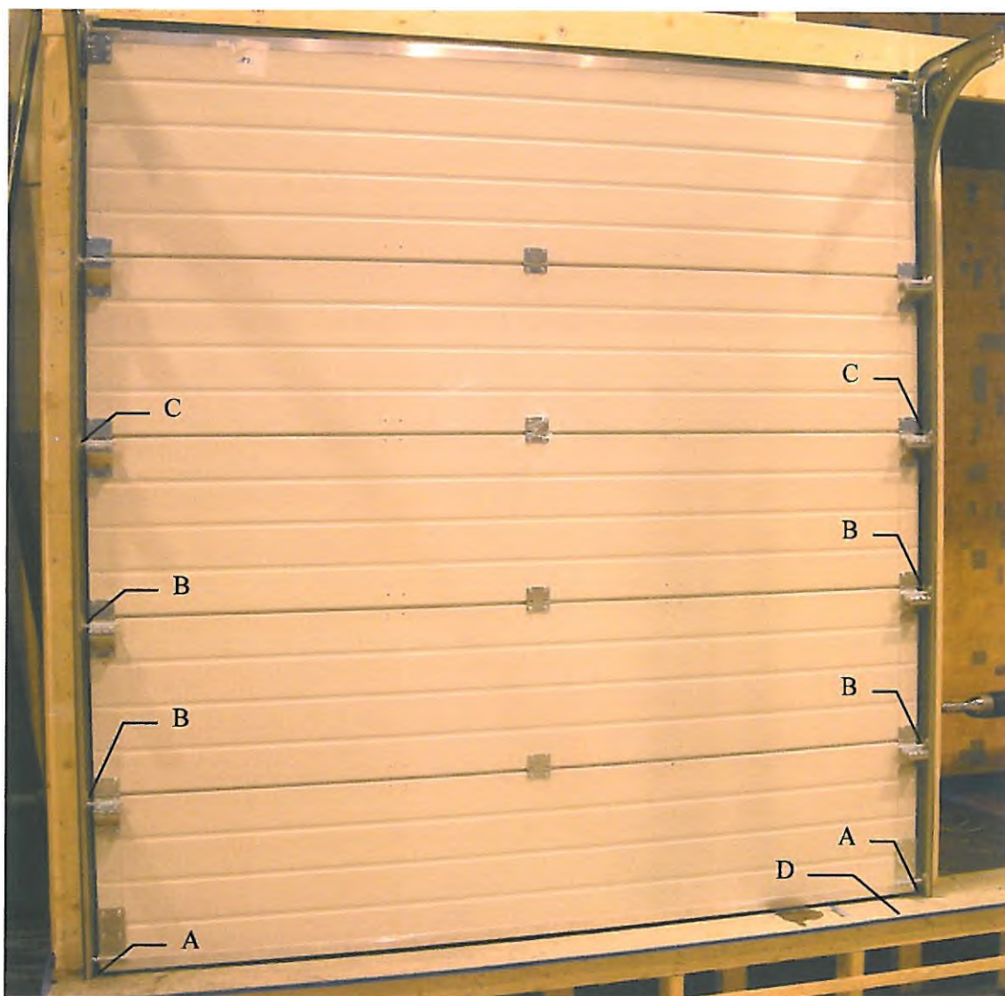
Figure 1. The door as seen from inside.
