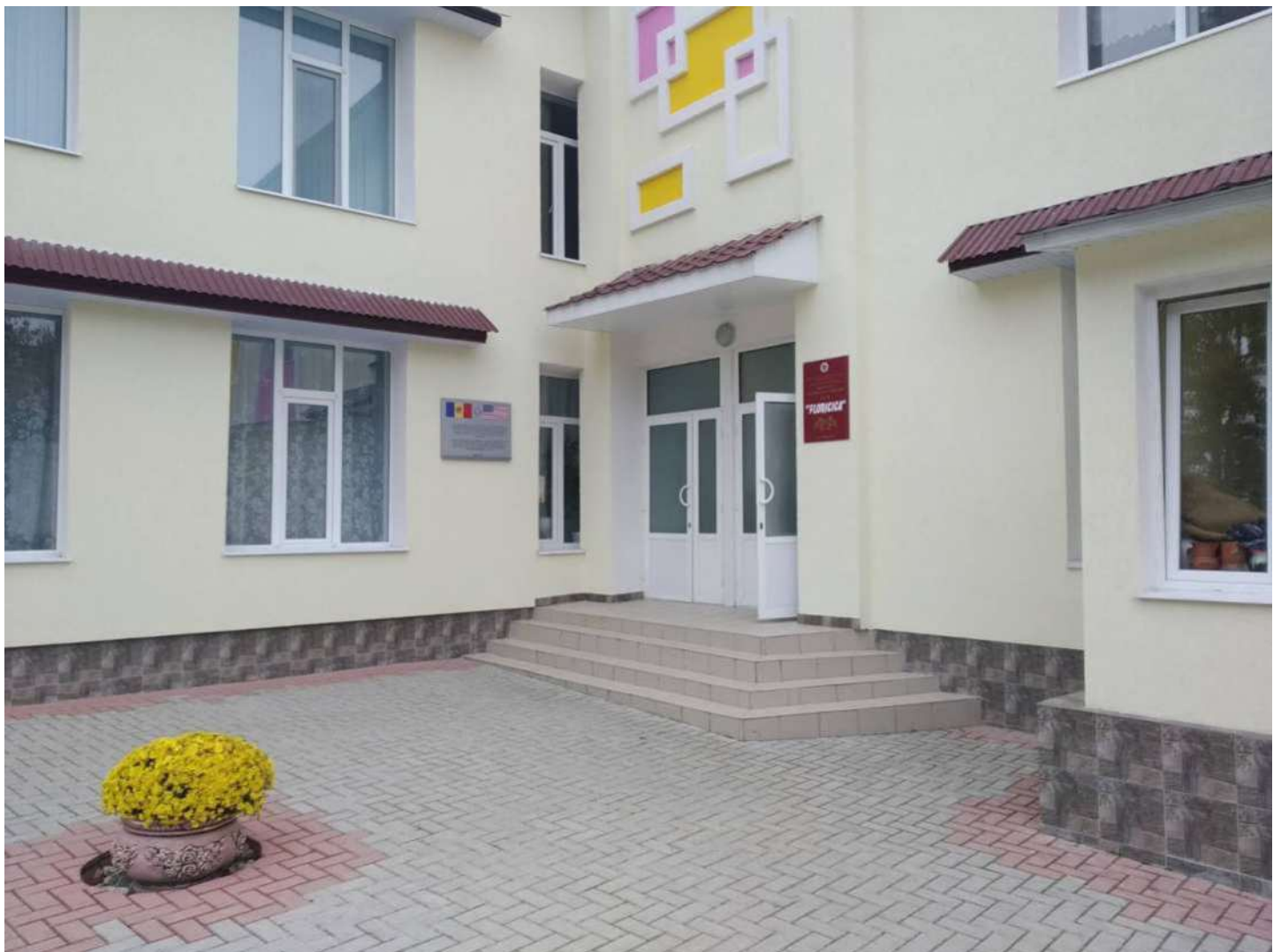
Picture from recently completed kindergarten renovation project in Moldova (Drochia). Typical pavement required around the new building for minimum of 1,000 m 2 including all CLIN's. Note also acceptable façade finishes and commemorative plaque.
