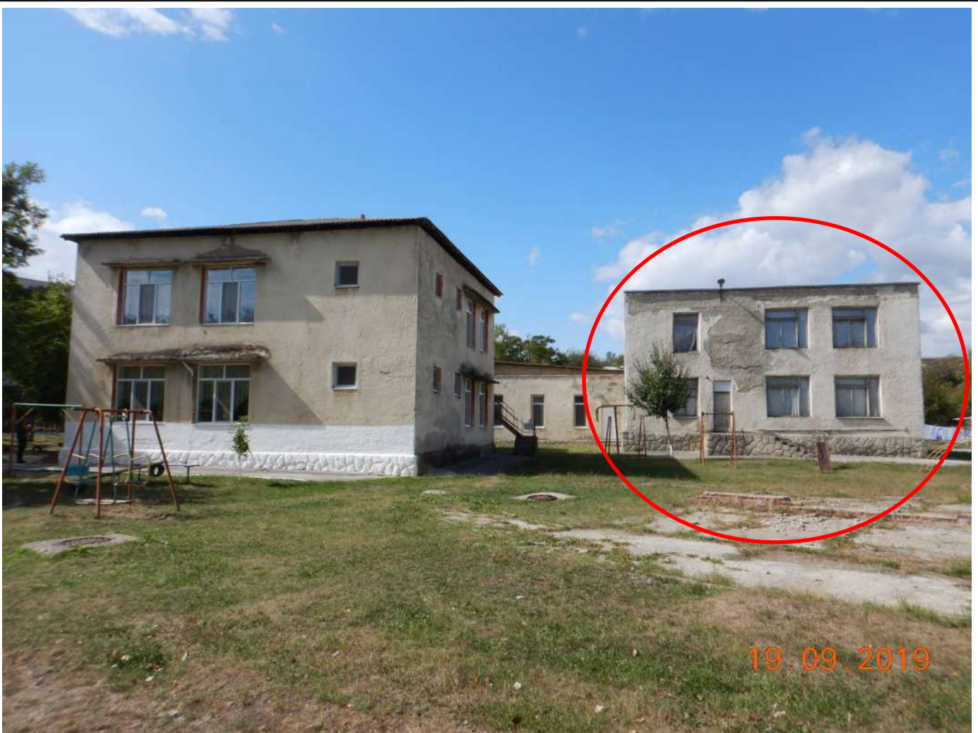
In red: north-east block to be demolished. Rest of building to remain.
