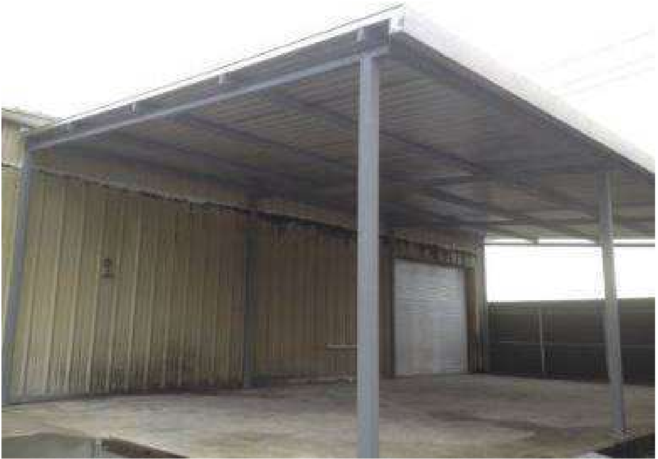
Metal canopy attached to a building, conceptually similar to the one required by our contract.
