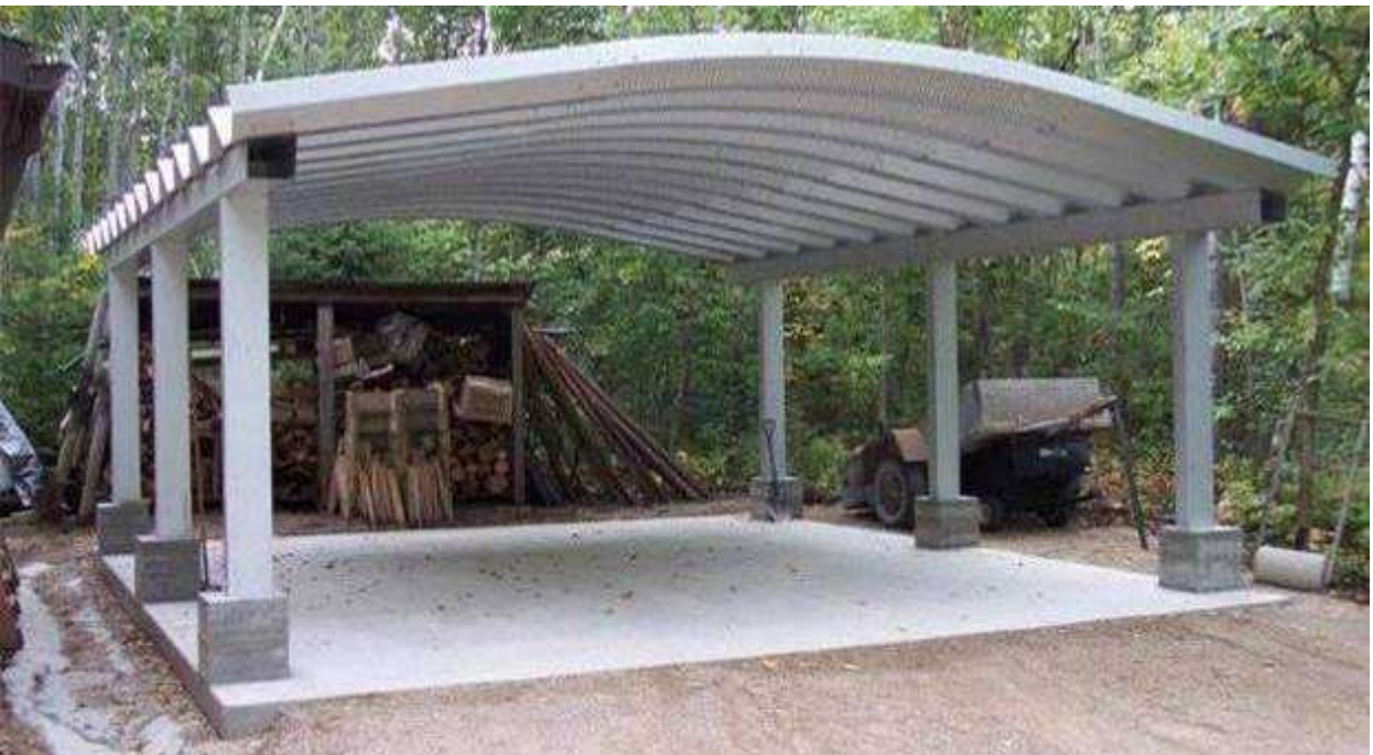
Self-standing canopy provided by NAVFAC in Ukraine. Similar design is acceptable, with only 3 columns separate from the building facade
