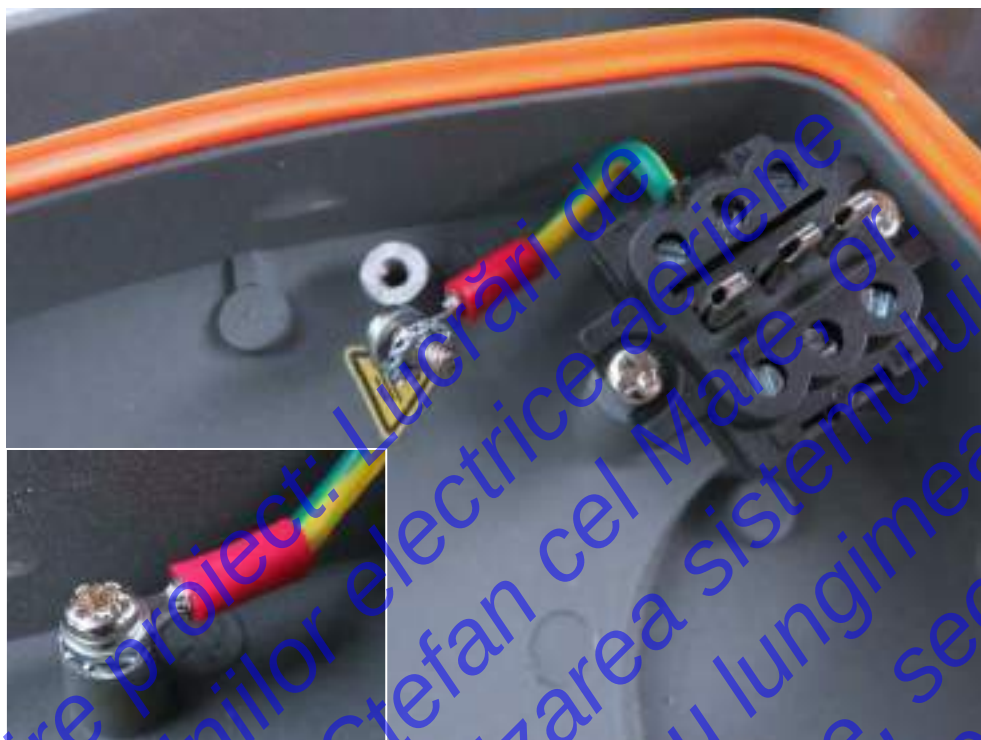
M60W36L505057CRI70KHP10D6I60TDD2CLI metal cover earthing
