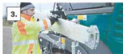
Fix the central beam in position.
