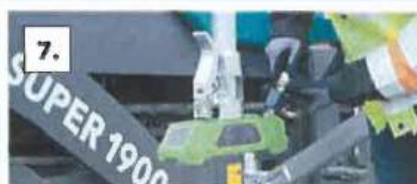
Route cables and connect sensors.
