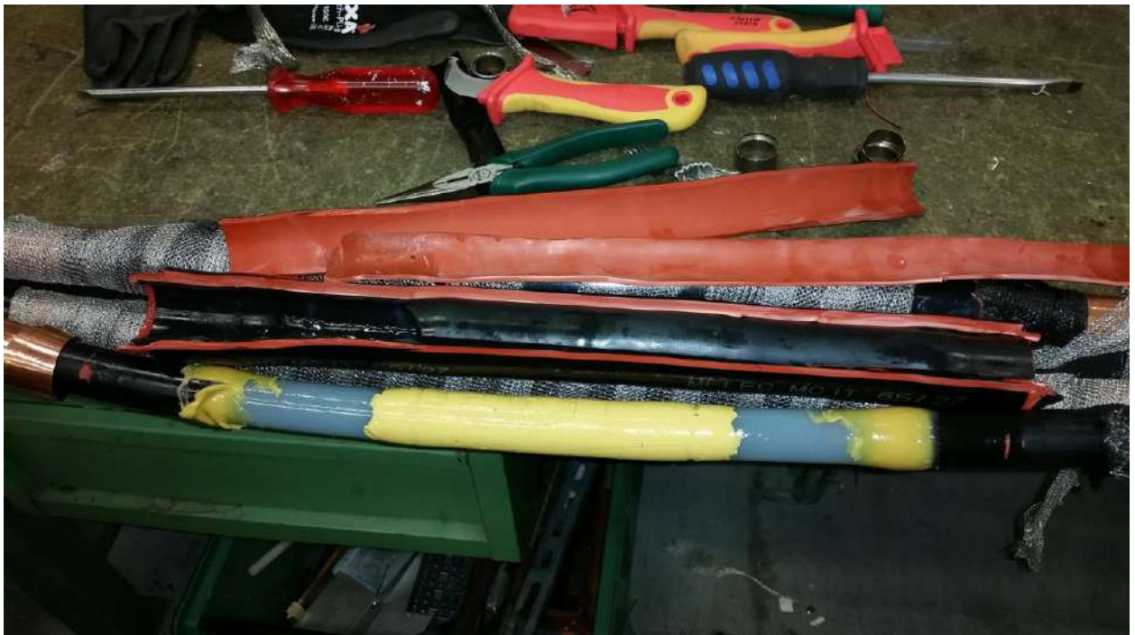
Electrical field stress control
