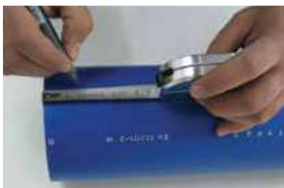
Measure and mark the pipe
