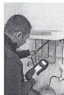
Ambient CO checking
