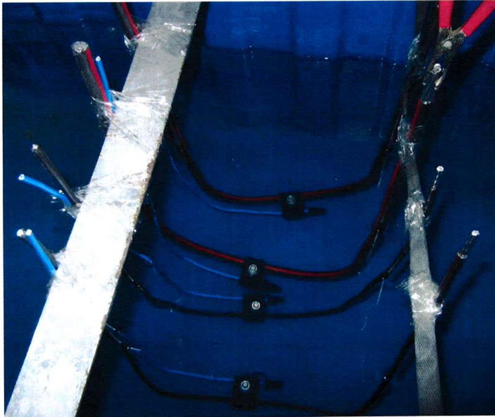
Fig.1 – IPC during the testing
