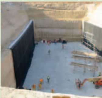
Dubai International Airport, UAE, Tunnel tanking
