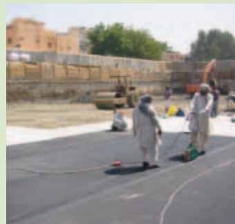
Arab National Bank in Jeddah, Saudi Arabia, Basement tanking
