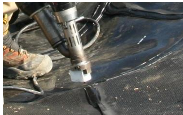
Extrusion welding
