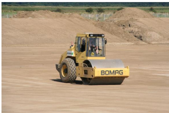
Subsoil preparation for the following day's lining progress
