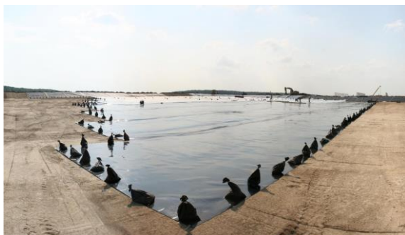
Temporary loading with sand bags
