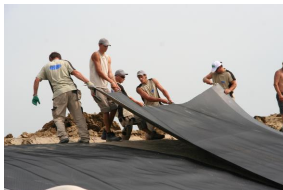
Installation on slope
