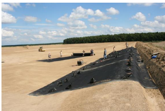
Seams parallel to the slope
