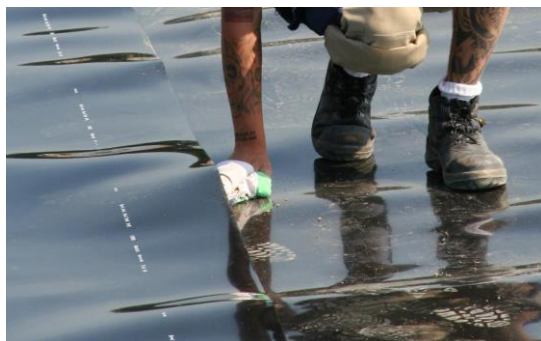
Cleaning of the seam area
