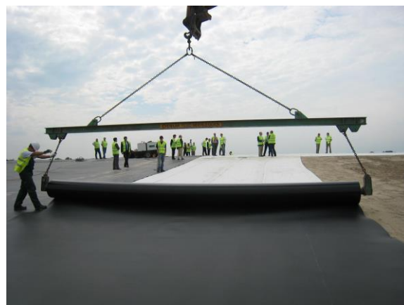
Sealing of long slopes
