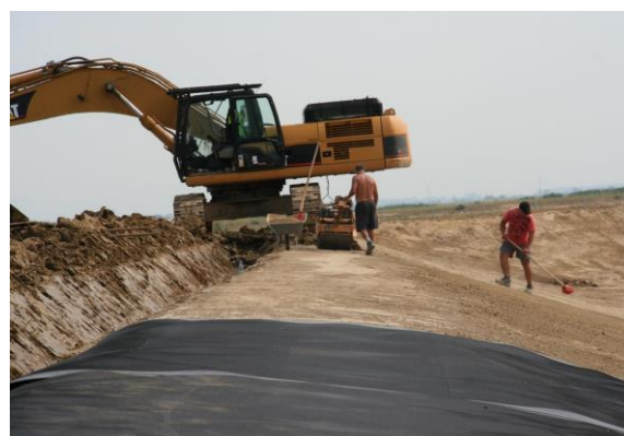
Repair of small defects
