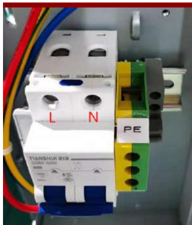
Figure2-4 Single phase-three-wire connection
