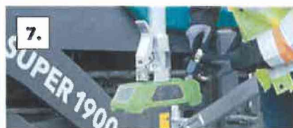
Route cables and connect sensors.
