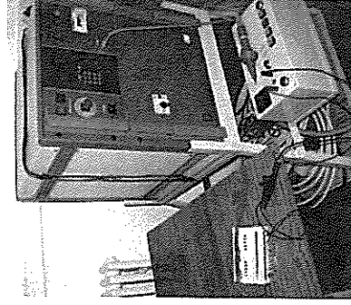
Figure 4 Dielectric strength test
