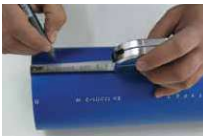
Measure and mark the pipe
