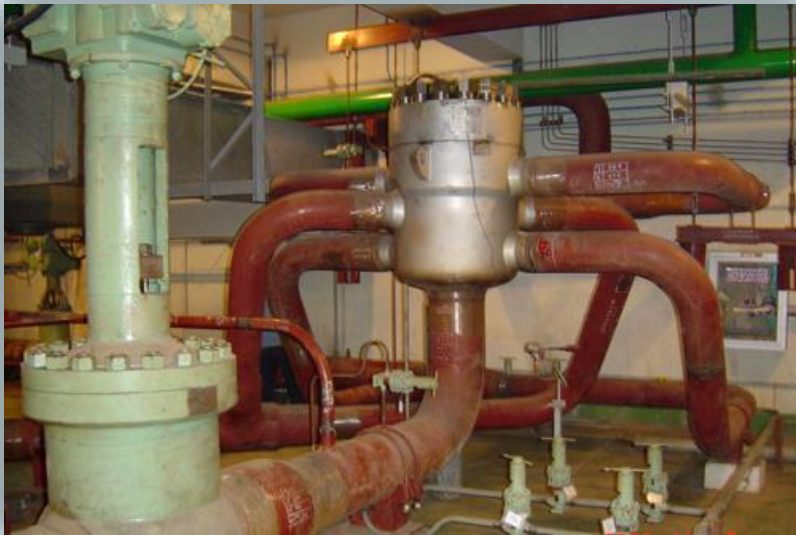
General view of the assembled CPHTD pump unit 850–400 A before installation of thermal insulation
