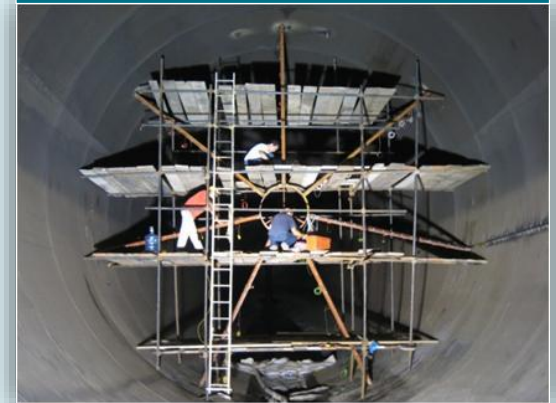
Installation of hydrometric propellers in the penstock
