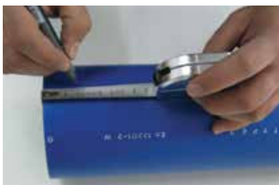
Measure and mark the pipe
