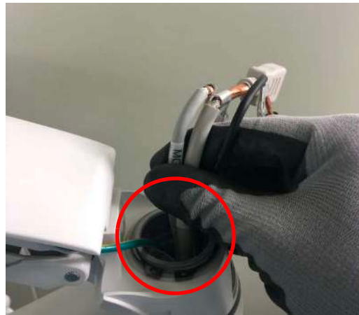
Figure 8-256 Extracting 3 monitor cables
