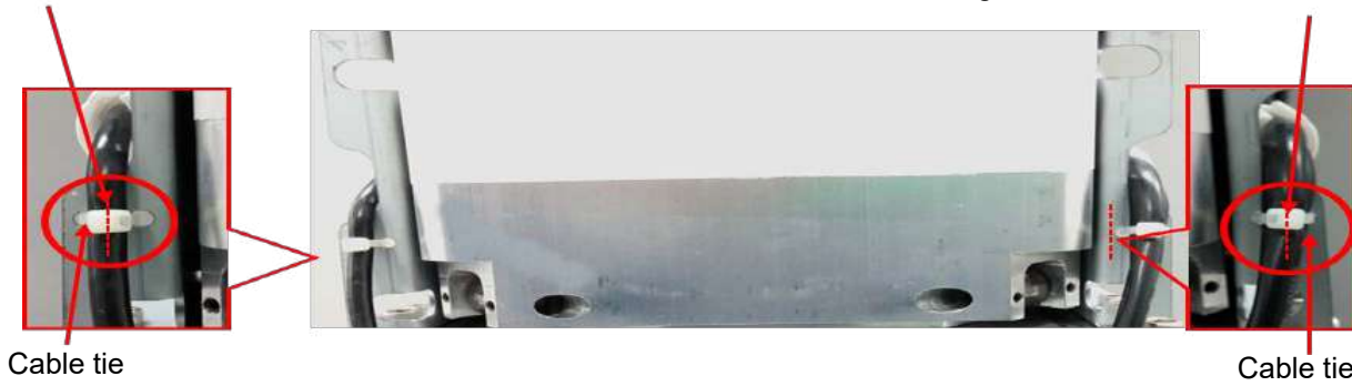
Figure 8-265 Tie cables with the ties through the holes
