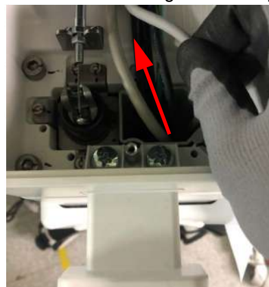
Extracting 3 cables through the hole
