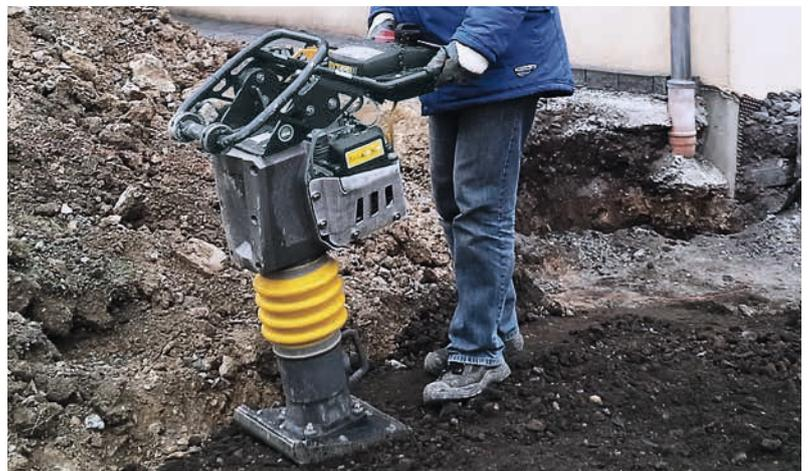
\*BOMAG tampers with Honda GXR 120 petrol engines (**BT 60** and **BT 65**) can also be used in trenches deeper than shoulder height and at least 1.5 m wide. Further information at: [www.bgbau.de](http://www.bgbau.de) (BG Bau, Deutschland, 2015).
