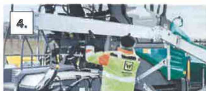
Suspend the extension beam.
