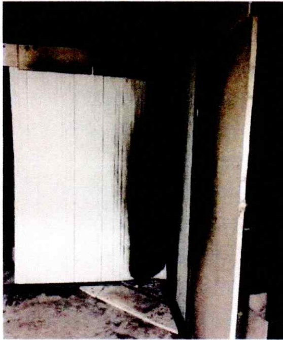
Photograph 3. Long wing detail of Sample 1 (After test)
