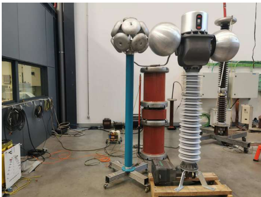
Power frequency and partial discharge test
