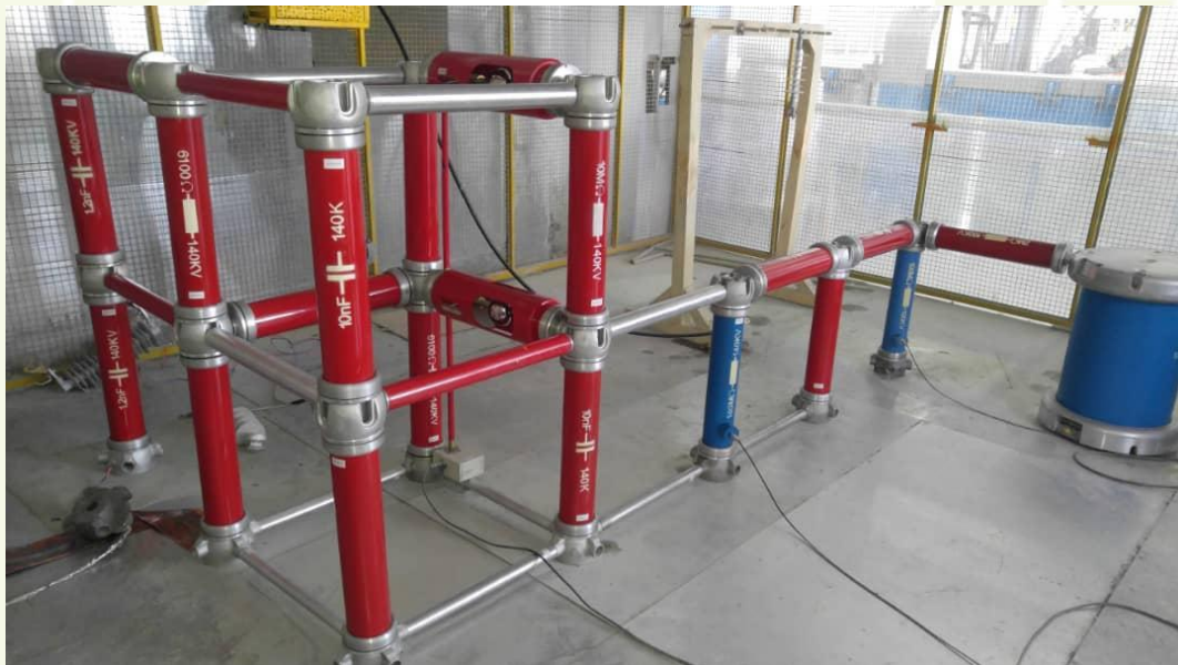
Figure 10: Equipment of Lightning Impulse Voltage Test (Date of test: 26-November-2024)
