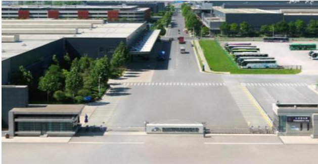
Shibalihe Plant Area
