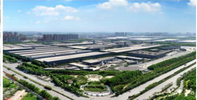
New Energy Bus Plant Area
