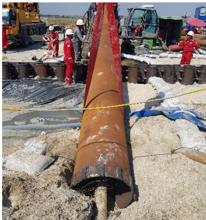
Instalare tub protector de inceput
