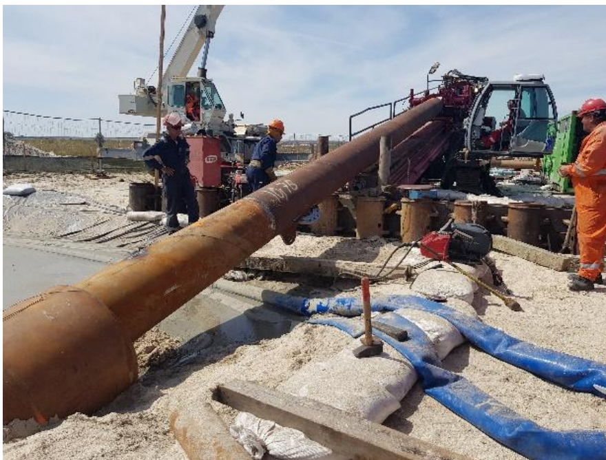
Exemplu instalare centralizator DN500 mm in tub protector DN800 mm
