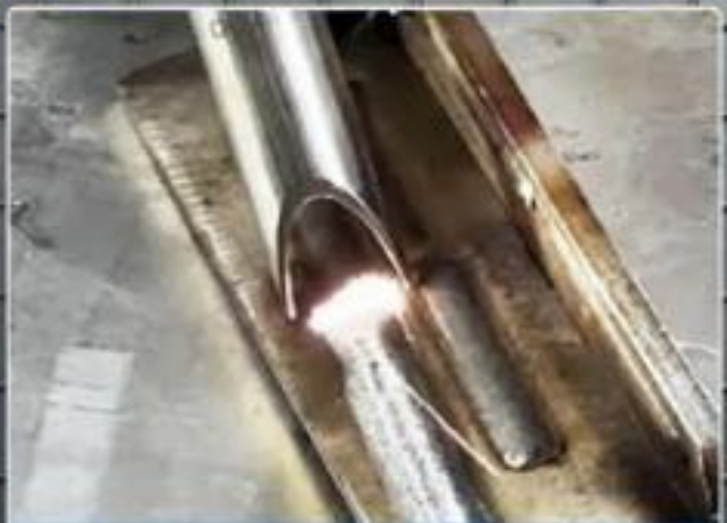
4 WELD SEAM CLEANING
