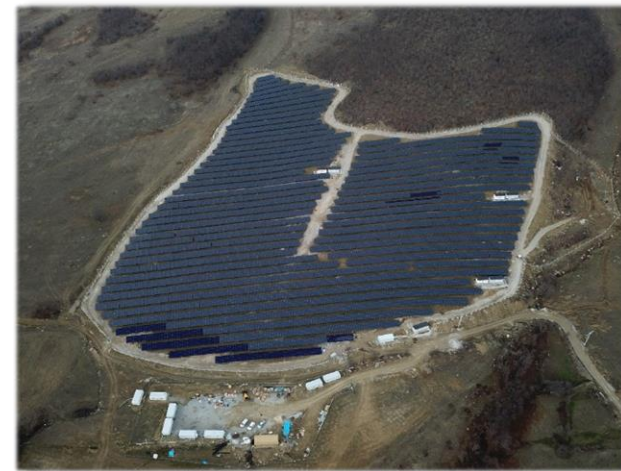
1198 kWp Solar Power Plant, Samsun / TURKIYE
