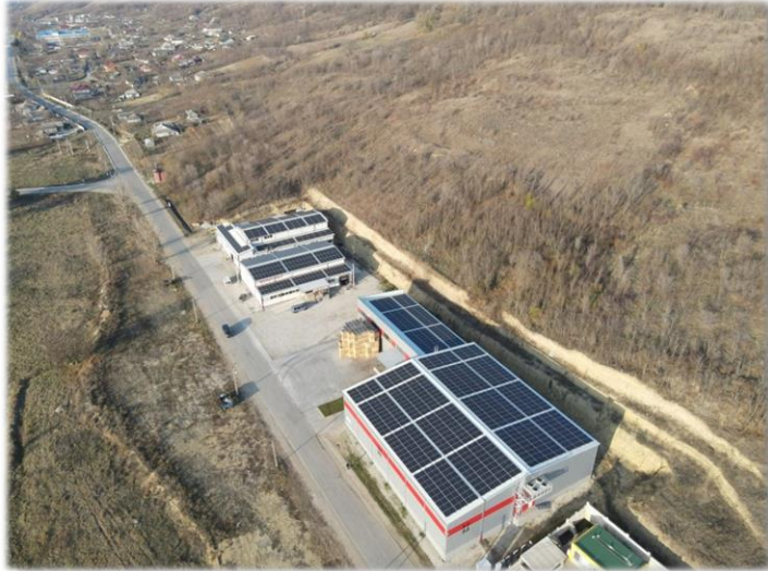
527 kWp Rooftop Solar Power Plant, Şişcani / MOLDOVA
