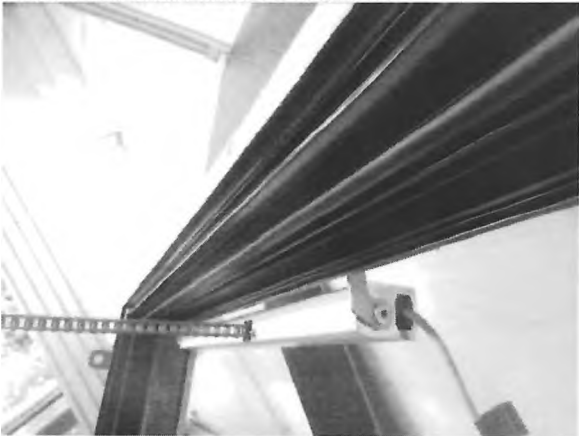
Picture 9 Connection chain drive to frame
