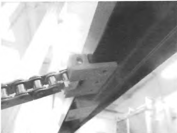
Picture 7 Connection chain drive to casement
