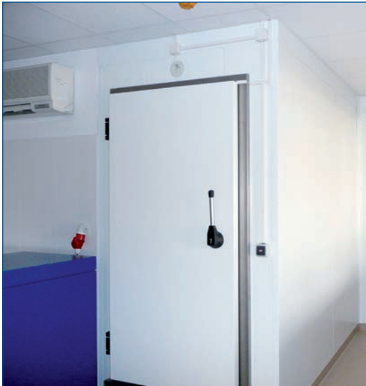
Cooling and freezing rooms for storing biological materials and blood plasma at temperatures down to -80 °C.
