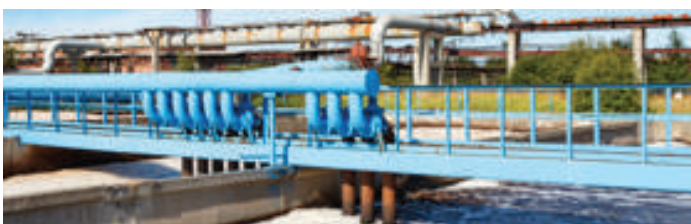
Waste Water Treatment Plant
