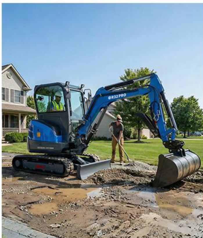
REPAIR A DRIVEWAY
