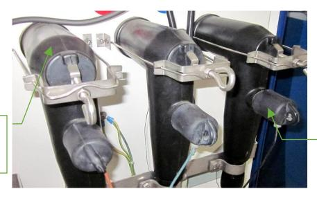
MV screened separable connector
