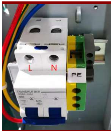
Figure2-4 Single phase-three-wire connection
