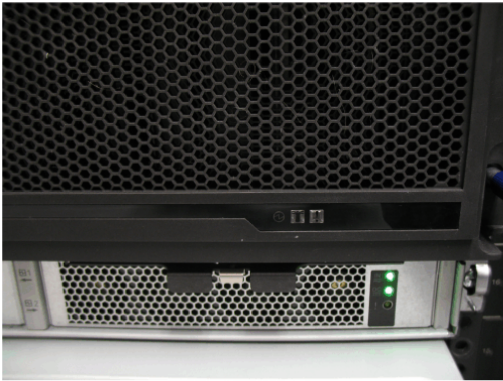
Figure 149. Fascia removed from the PSUs
