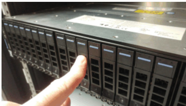
Figure 71. Completing the drive installation
