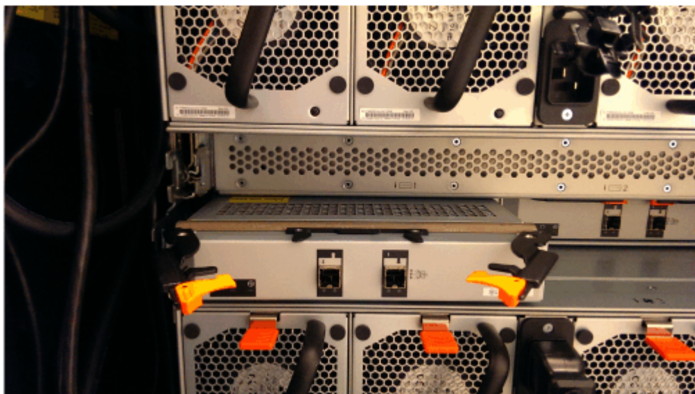
Figure 160. Removing the expansion canister
