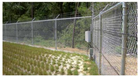
APACHE FIBER is a perimeter protection system with optical fiber suitable for the detection of intrusion fence. It uses optophonic technology for the detection of all those typical of intrusion attempts like climb, cut or break through the fence.
